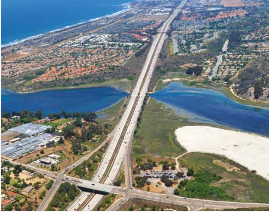
FIGURE 2 – THE ORIGINAL I-5 BRIDGE OVER BATIQUITOS LAGOON UTILIZED SUBSTANTIAL FILL, ARTIFICIALLY NARROWING THE LAGOON CHANNEL AND CREATING IMPACTS TO BOTH WETLAND HABITATS AND NEIGHBORING PROPERTIES. (PHOTO: CALIFORNIA DEPARTMENT OF TRANSPORTATION)
